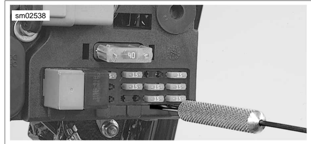
Figure 8-2. Removing Relay/Fuse Panels
